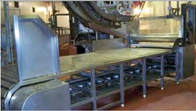
Further view of the all s/s unloading table from the primary de-hairers and re-shackling line and inspection table.
