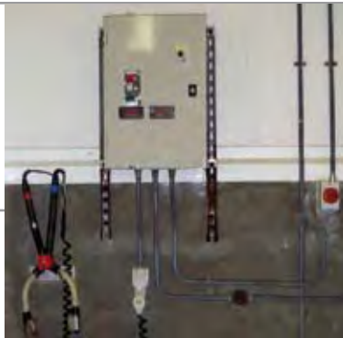
Manual stunner in holding area.
