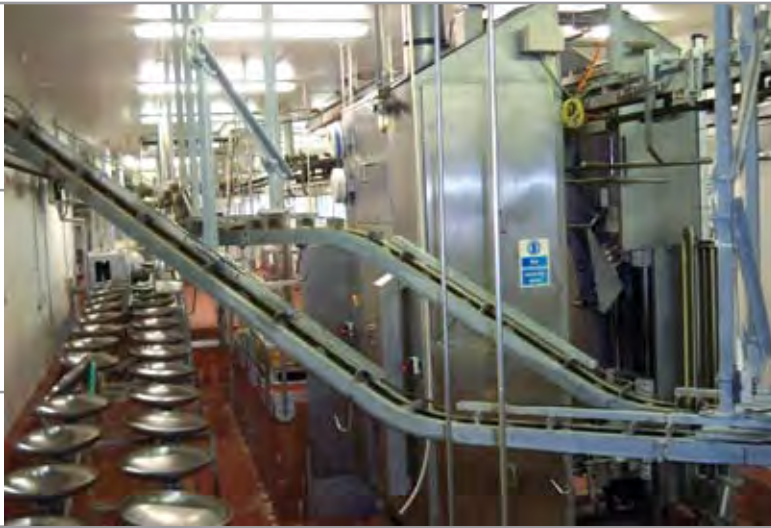
Overall view of the fully automatic pig splitter and offal tray system.
