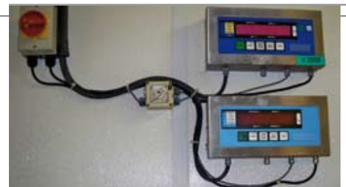
Part of the overhead scale system with digital readout.
